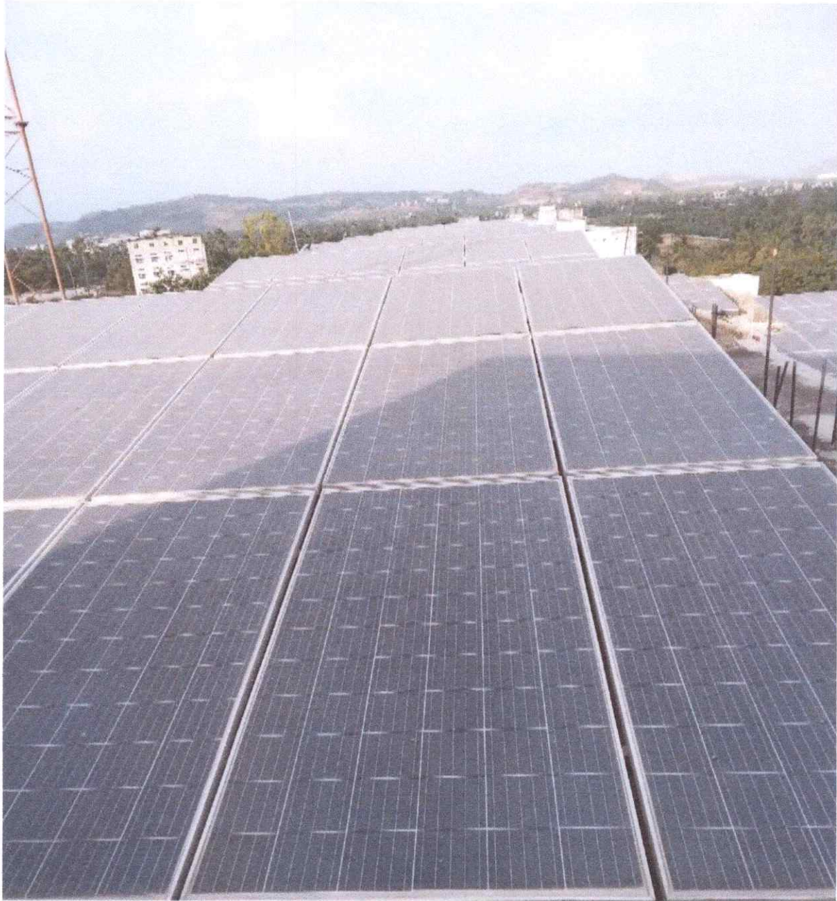
Solar panels were installed on the rooftops
